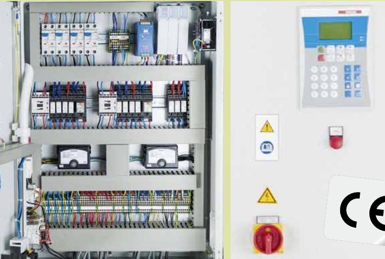
Control cabinet, control voltage 24 V, juice pump, SPS for automatic control and regulation of all functions
